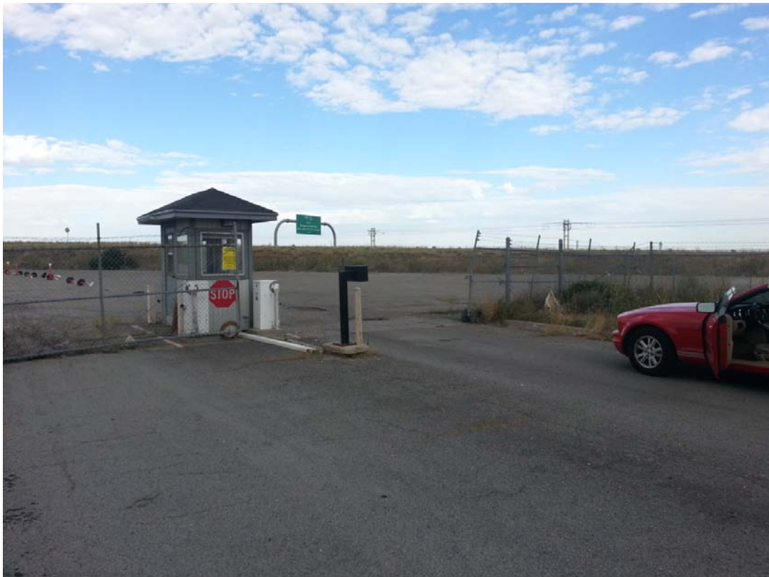
Former Continental Airlines Reservation Center site between North Temple on-ramp and I-80 at 2400 West
